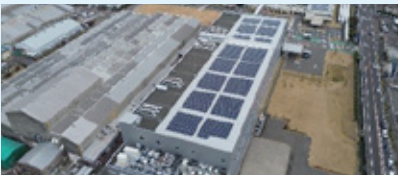
Solar power generation equipment at Suzuka Factory
