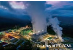
Geothermal power generation
