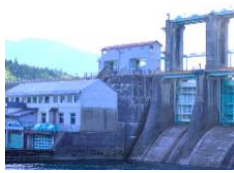
Hydropower generation facilities
