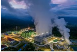
Geothermal power generation facilities
