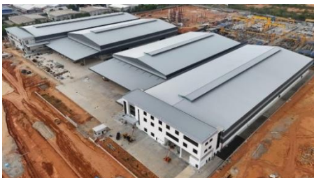
The new production building under construction (Malaysia Factory)
