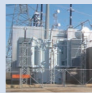
High-capacity transformers
