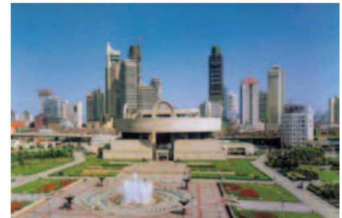
Sites where high reliability and easy maintenance are required (Public facilities such as museums, airports, etc.)
