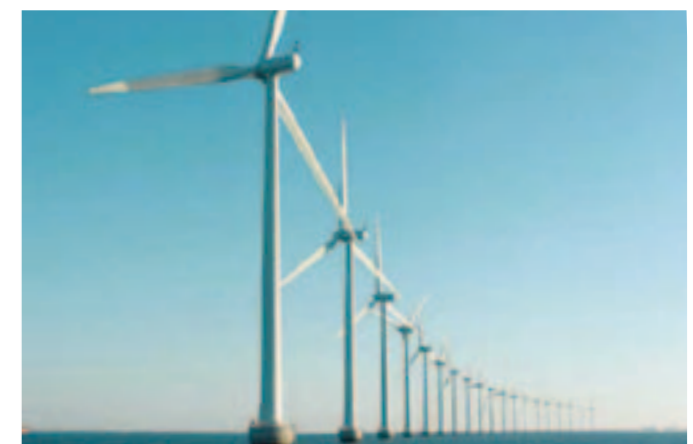
Wind power site
