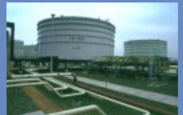
A plant of Japan Underground Oil Storage Co., Ltd.
