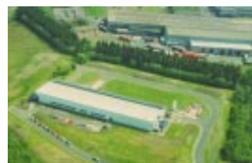
Fuji Electric (Scotland) Ltd. (photo by Graeme Macklin)
