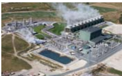
Fuji Electric delivered the world's largest-capacity* (140MW) geothermal power plant to the Nga Awa Purua geothermal power station in New Zealand.
