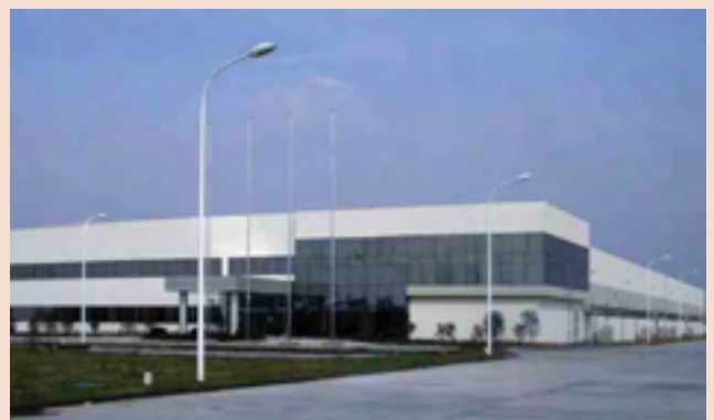
Wuxi plant (China)
