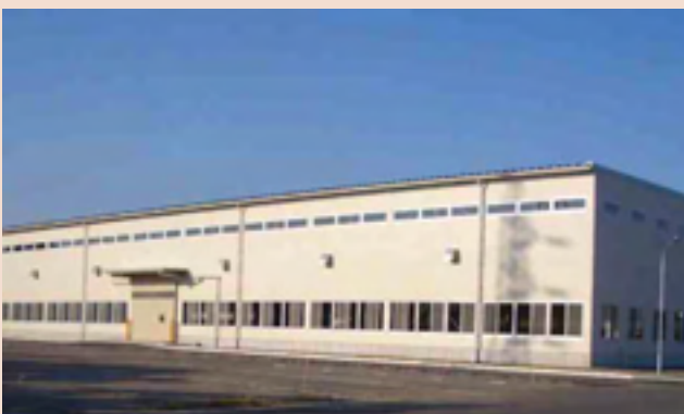
New testing facility at Suzuka inverter plant (completed October 2006)
