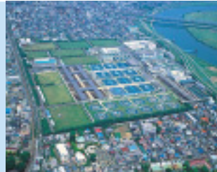
Water Treatment Systems
