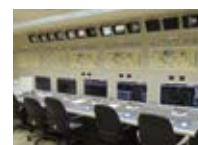
Plant monitoring and control system
