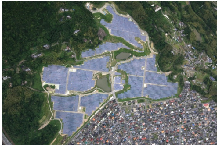
Mega solar plant in Hikari City, Yamaguchi Prefecture owned by Hikari Energy LLC EPC project with annual generation capacity of 14 MW completed in January 2017
