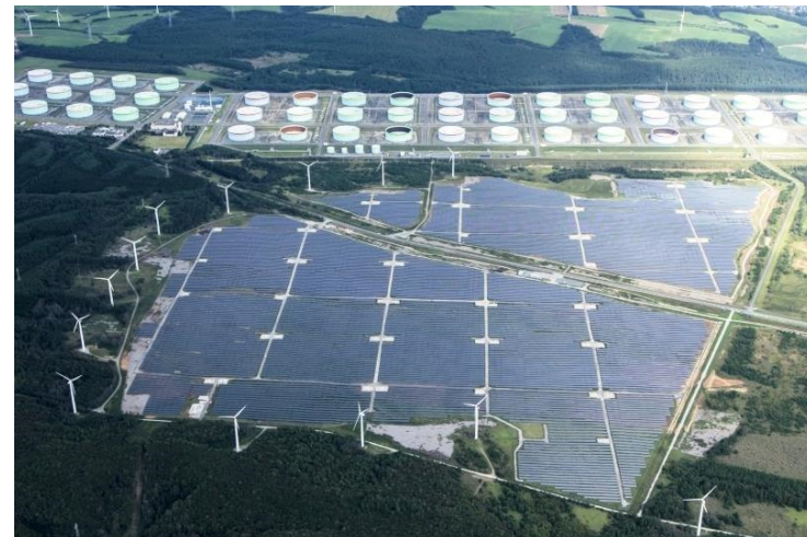
Kamikita Rokkasho Solar Power Plant of Mirai Power (Kamikita Rokkasho) Corporation (subsidiary of Sojitz Corporation) EPC project with annual generation capacity of 51 MW completed in March 2017
