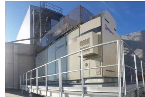
100 kW fuel cell for cold storage warehouse of Wolf Butterback KG (completed in 2016)
