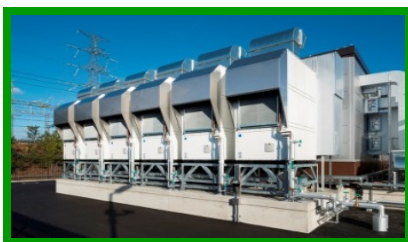
Indirect outside air-conditioning
