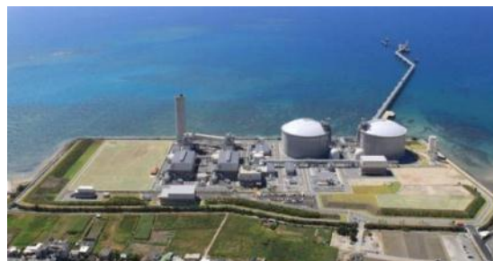
Okinawa Electric Power Company, Incorporated Yoshinoura Thermal Power Plant (Combined-Cycle Power Plant)
