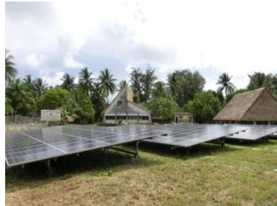
Kingdom of Tonga Microgrid for Isolated island (Scheduled for completion in 2015) • PV panels (1 MW) • Electricity storage system for grid stabilization • PCSs (500 KW × 4) • Complete high-voltage switchboard system • Grid monitoring and control system
