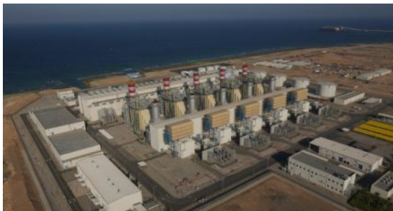
SUR IPP (Combined-Cycle Power Plant / Oman)
