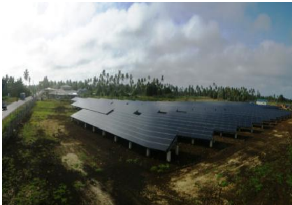
Kingdom of Tonga Microgrid for Isolated island (Scheduled for completion in 2015) • PV panels (1 MW) • Electricity storage system for grid stabilization • PCSs (500 KW × 4) • Complete high-voltage switchboard system • Grid monitoring and control system
