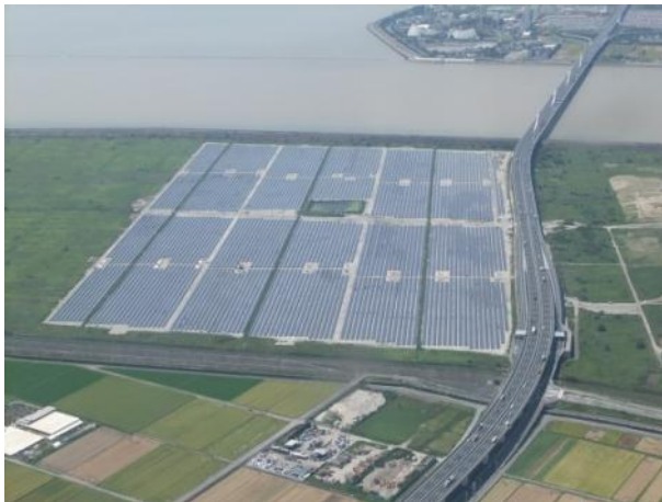
Kisozaki reclaimed land mega-solar (49MW) (Scheduled for completion in 2015) (Mie Prefecture and Aichi Prefecture)
