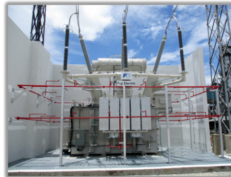
Asia business (Thailand /transformers)
