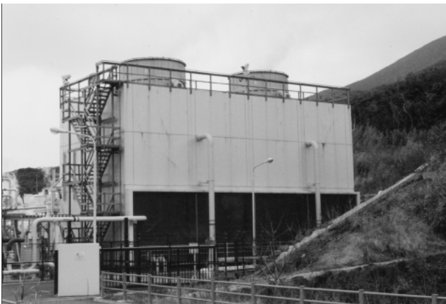
Fig.11 Exterior view of the cooling tower
