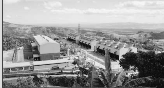
Malitbog 3x77.5MW geothermal power plant, VGPC, Philippines
