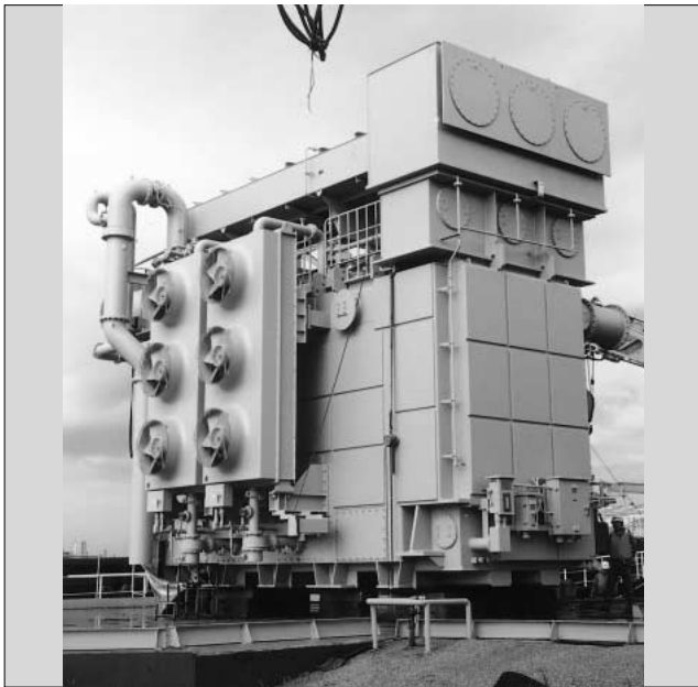
Fig.8 Shipping of the transformer with the steel plate dampers mounted
