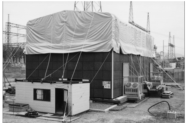
Fig.8 Dust-proof and air-conditioned building
