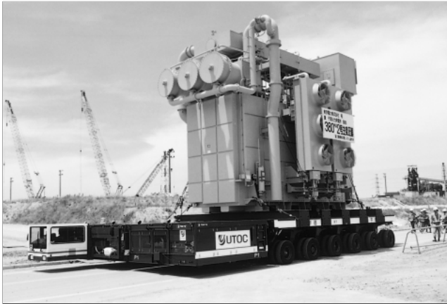
Fig.2 Main transformer being transported in a complete bank
