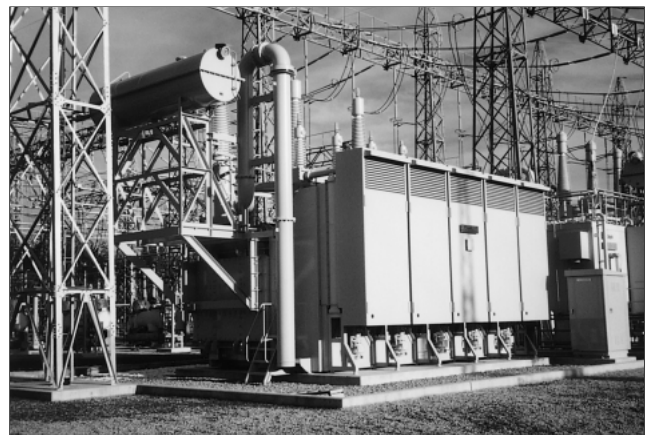
Fig.9 Onsite completed FATRAS
