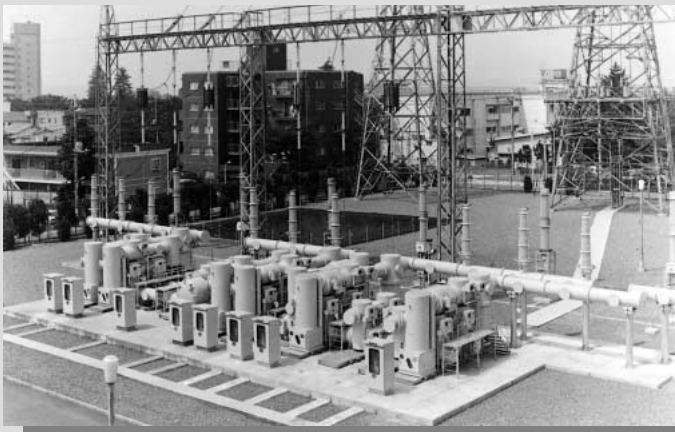
170kV three-phase-encapsulated GIS
