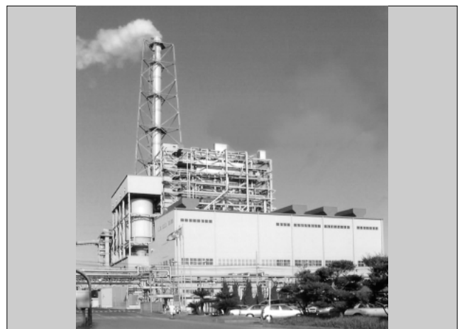
Fig.2 View of the entire UBE Power Center Plant
