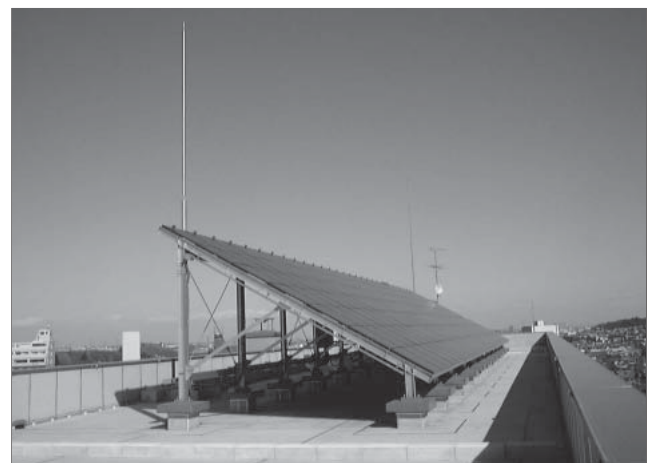
Fig.3 Onsite installation of solar cells
