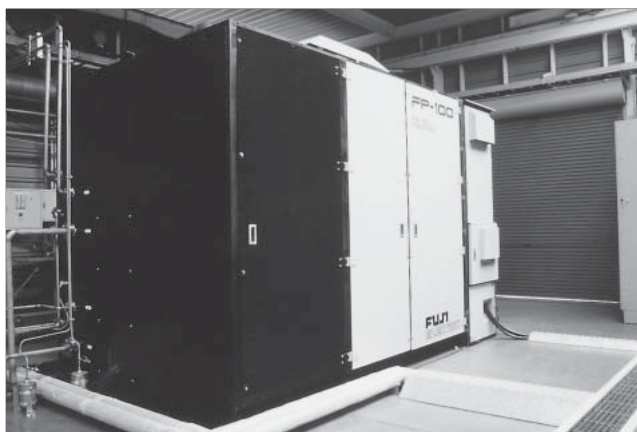
Fig.1 External appearance of a 100 kW PAFC
