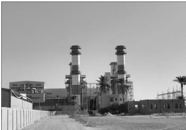
Fig.49 GECOL Benghazi combined cycle power plant
