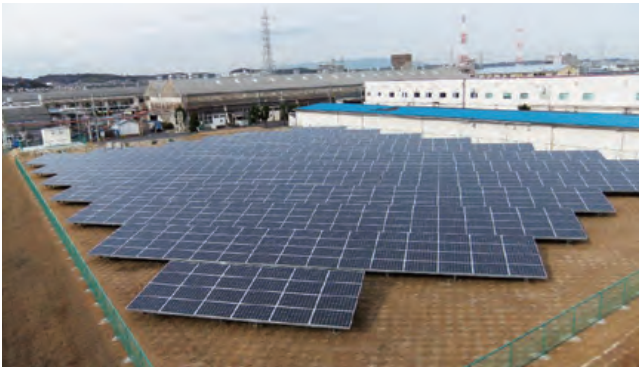
Solar power generation system introduced at a Smart Factory Initiative model factory (Mie Factory)
