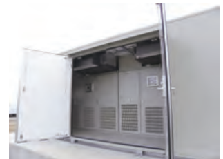
Power conditioners in an outdoor container at the Moji Power Plant
