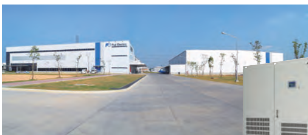
Fuji Electric Manufacturing (Thailand) Co., Ltd.
