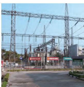
Industrial park substation
