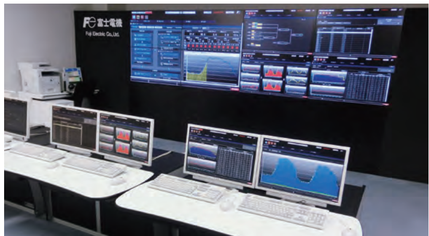
Cluster Energy Management System (CEMS)
