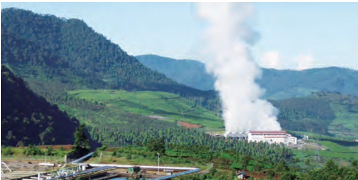
Wayang Windu Geothermal Power Station (Indonesia)
