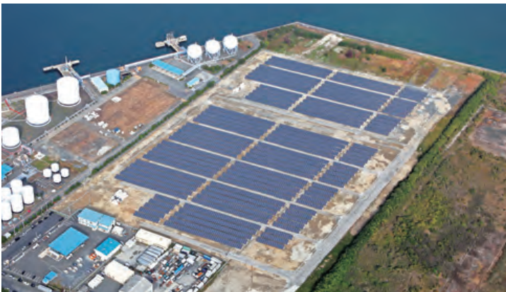
Idemitsu Kosan Moji Power Plant
