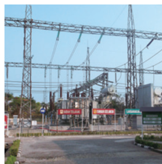
Industrial park substation
