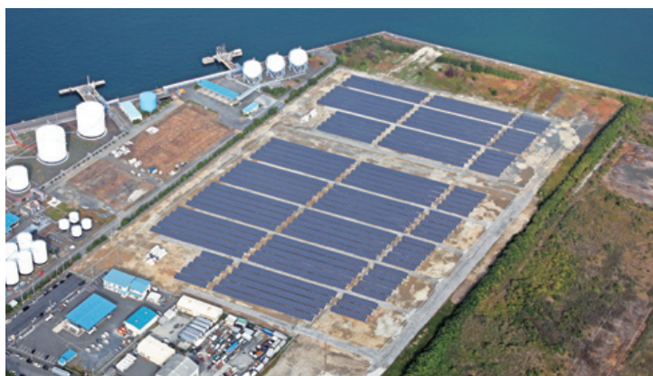
Idemitsu Kosan Moji Power Plant
