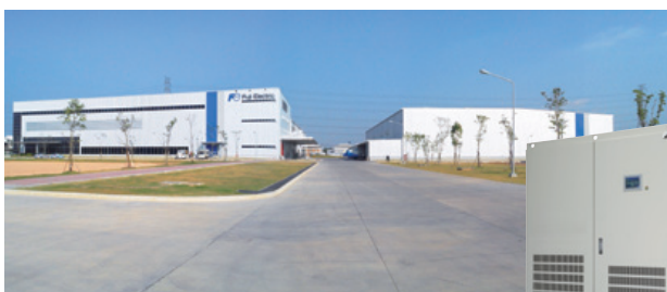
Fuji Electric Manufacturing (Thailand) Co., Ltd.
