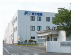
Fuji Electric acquired a subsidiary of Renesas Electronics Corporation and established Fuji Electric Tsugaru Semiconductor Co., Ltd. with a view to enhancing its production capacity for power semiconductors and dispersing risk
