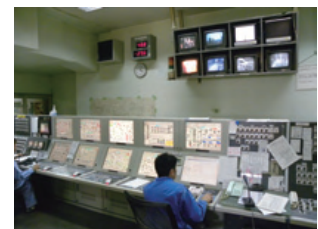
The production monitoring control system visualizes cement production processes
