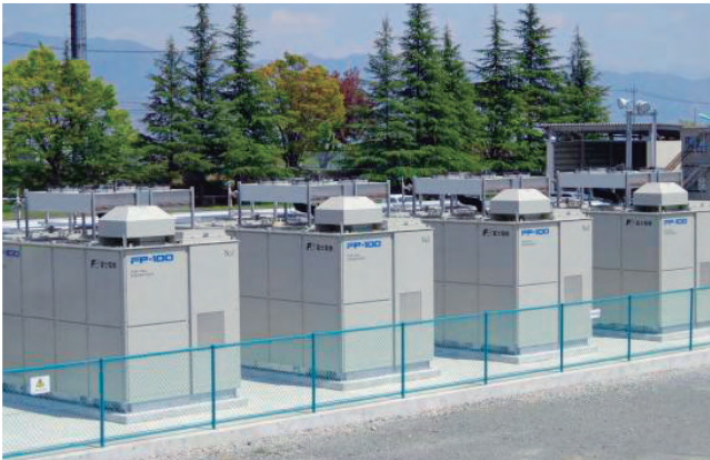
Fuel cells installed at the Yamanashi Branch Factory under the Smart Factory Initiative
