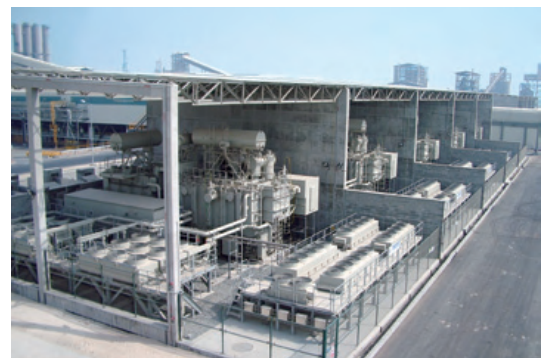
This photo at EMAL's aluminum smelting plant shows some of 12 S-Formers delivered for first-phase construction. Once six more S-Formers are delivered for the second phase, the smelter will be among the world's largest
