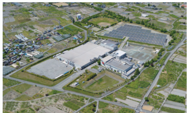
Start of processing and mass-production of 8-inch wafers for power semiconductors at the Yamanashi Factory
