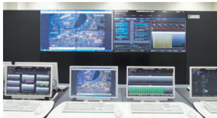
Cluster Energy Management System
