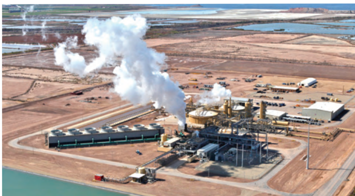
Hudson Ranch I Geothermal Power Plant (HRI): HRI and HRII each generate enough power to serve 50,000 homes in the Southwestern region of the U.S.
