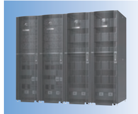
Uninterruptible power supply systems (UPSs)
